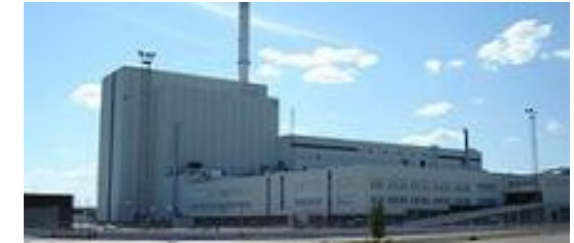
Kärnkraftsverket Forsmark Power up rate, reinforcement of cooling water building
