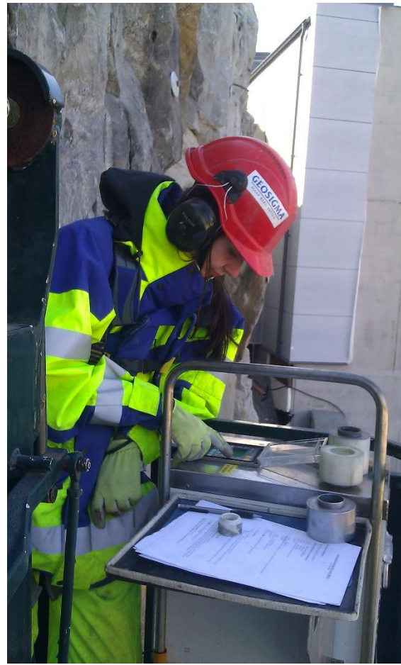
Geosigma provides personnel, equipment and performs pull-out tests.
